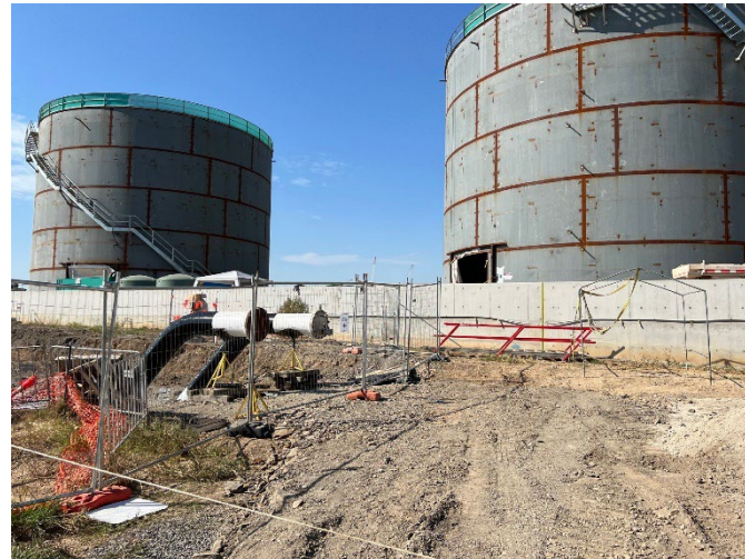
New fuel facility at Western Sydney Airport
